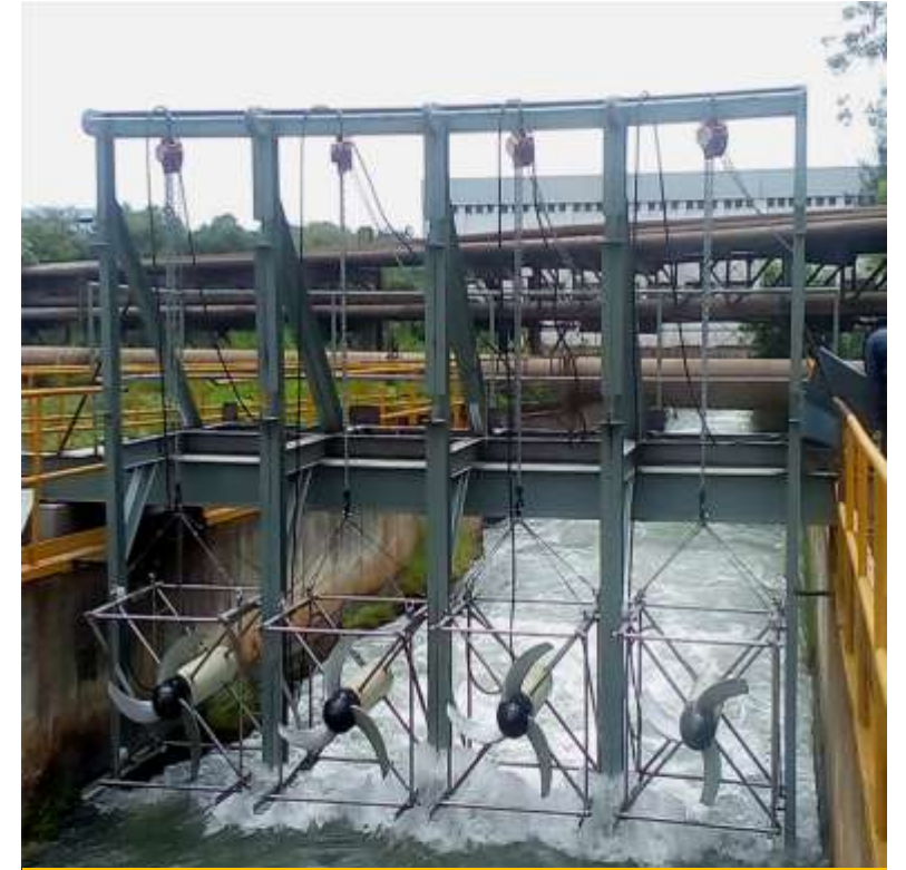
HYDRO KINETIC TURBINES
